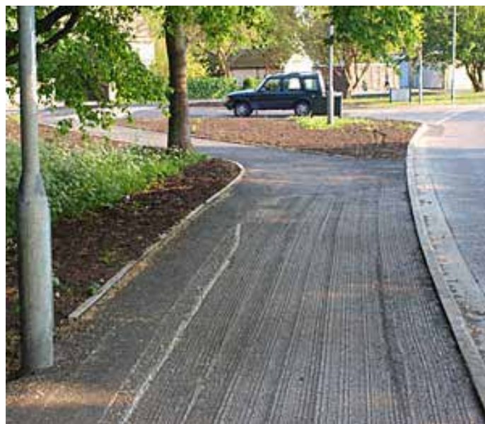
Cottenham–Histon cycle path – an example of good practice. At crossings the path (shown under construction) leads away from the corner.
