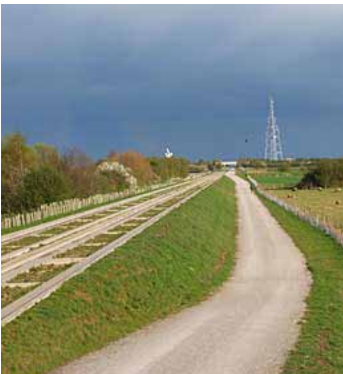
The guided busway maintenance track between St. Ives and Over.
