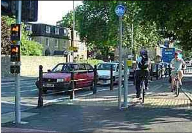
*The north side of Gonville Place Crossing. Many cyclists cannot make the sharp left turn without veering onto the opposite side of the two-way cycle path.*
