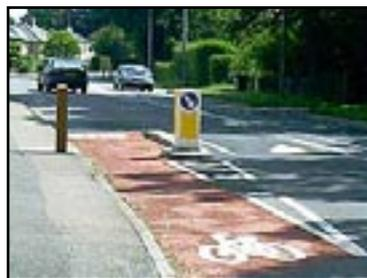
*The final construction has a 1.3 m cycle escape.*
