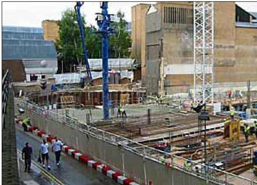
The first concrete is poured for the floor of the cycle park at the Grand Arcade development: Corn Exchange Street is in the foreground, Lion Yard in the background. The street entrance will be at the Guildhall end, near where the workman on the road is bending over.
