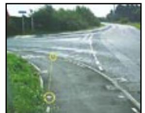
*At junctions following the apparent path of the catseyes could be a recipe for disaster.*
