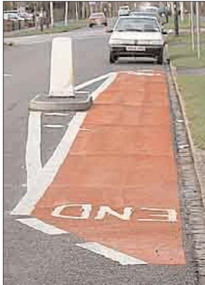
The traffic calming scheme on Radegund Road is now complete. It consists of a raised table and a series of narrowings where cars have to give way to oncoming traffic. Short lengths of cycle lane allow cyclists to by-pass these narrowings in both directions. Unfortunately these are much too short (as we repeatedly said during the consultation) allowing cars to park close to the narrowings, forcing cyclists to weave in and out.
