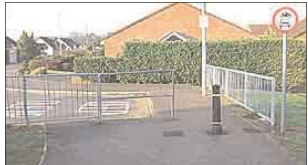
A chicane at the Cherry Hinton side of Fulbourn Old Drift has been widened, but there is still no dropped kerb on the other side.
