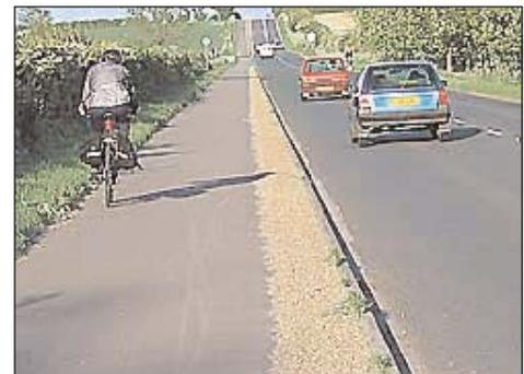
Instead, the cycle track alongside Fulbourn Road was laid with a miserable bit of glued-on shingle along the edge which reduced the useful width from just about OK to narrow, and leaves the path permanently covered in little bits of gravel – just what the cyclist needs!
