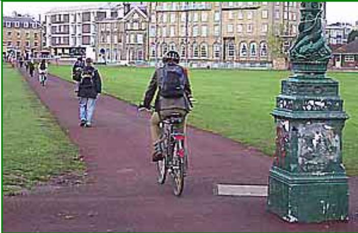
*The pedestrian- and cycle-path from Mill Road to Regent Street has been resurfaced in red, at last obliterating a confusing central white line that was left over from a long-abandoned scheme to segregate cycles and pedestrians. The result is a noticeable improvement on the previous pot-holed surface, but because this was a cheap and cheerful 'slurry seal' and not a full resurface, the result is still quite bumpy. This is one of the busiest cycle paths in Cambridge, and deserves better.*
