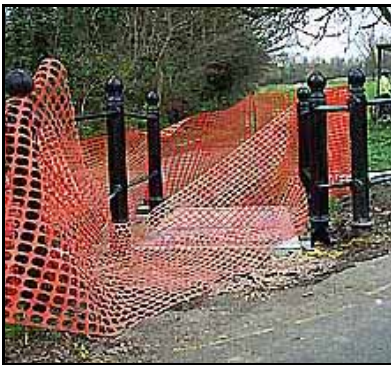
Cattlegrids are much better than pinch stiles, but take care to cross them at right angles, and don't brake or turn on them – they are very slippery when wet. This one is being installed on Trumpington Road.
