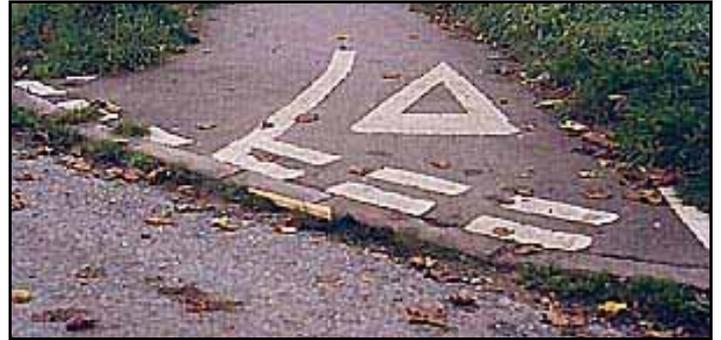
*This is a typical dropped kerb on Stapleford to Sawston route (white ruler is 24 mm x 300 mm) note also that vegetation has narrowed the path significantly and obscured its edge markings.*
