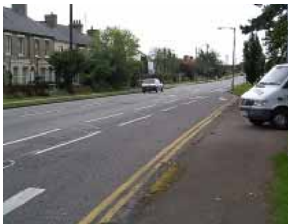
Shelford Road/ Trumpington High Street: The cycle lane should be made continuous and red
