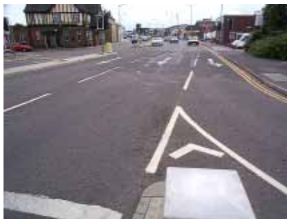
Newmarket Road/ Coldham's Lane
