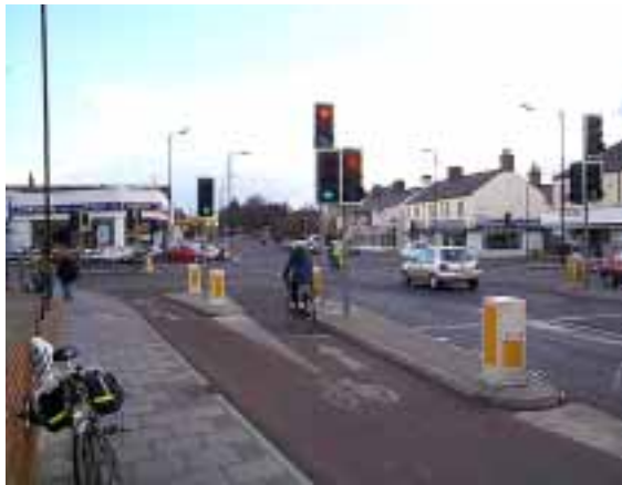
Separate signals allow cycles to go straight ahead from the left: Hills Road/ Cherry Hinton Road
