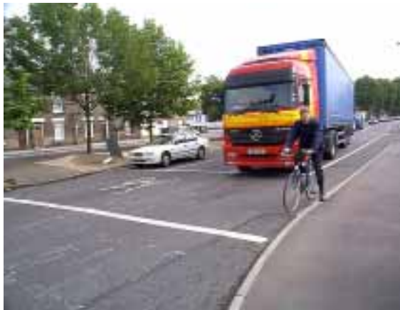
Red surfacing would make this advanced stop line even better: Newmarket Road
