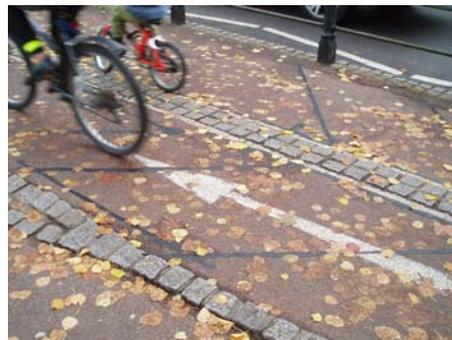
*Detector loops are still in place at the Gonville Rd crossing. They need connecting into the new system.*
