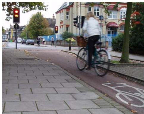
*Lyndwode Rd is a model cycle crossing, and is featured in "Cycle Friendly Infrastructure" <sup>8</sup>. The signals operate exactly as a normal road junction, relying solely on detector loops - no push buttons. Kerbs are also laid as a minor road junction.*
