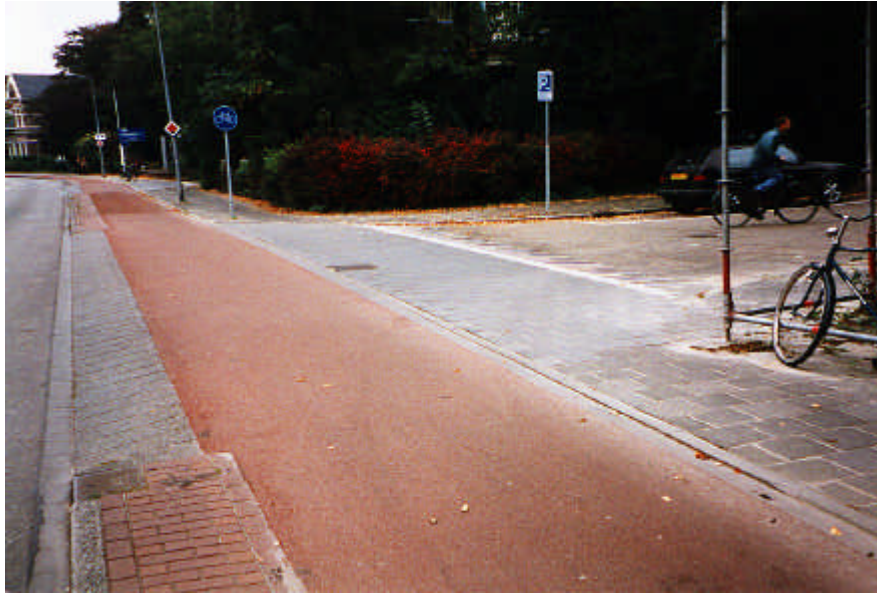
Groningen, Netherlands. (Give way lines in the Netherlands are a series of triangles, which can just be seen on the hump before the footway).
