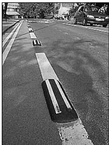
St Cross Road 6 , Oxford: cyclists receive protection from traffic but can easily join or leave the cycle lane. The separators should probably be slightly less protruding, for safety reasons.
