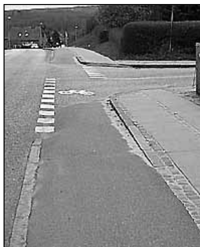
Århus, Denmark 5 : Cycle tracks merge smoothly with the road at minor junctions
