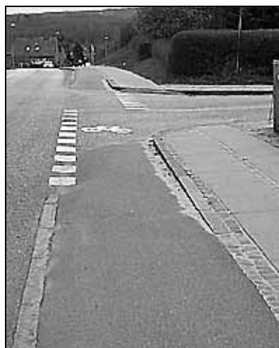
Århus, Denmark 7 : Cycle tracks merge smoothly with the road at minor junctions
