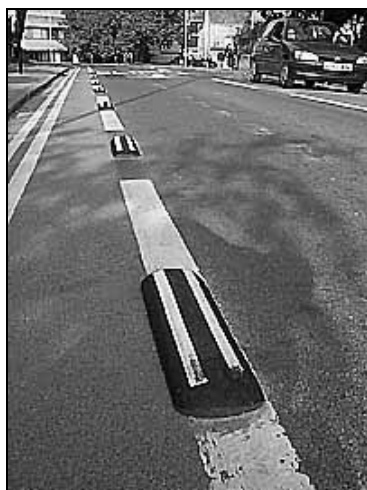
St Cross Road 4 , Oxford: cyclists receive protection from traffic but can easily join or leave the cycle lane. The separators should probably be slightly less protruding, for safety reasons.
