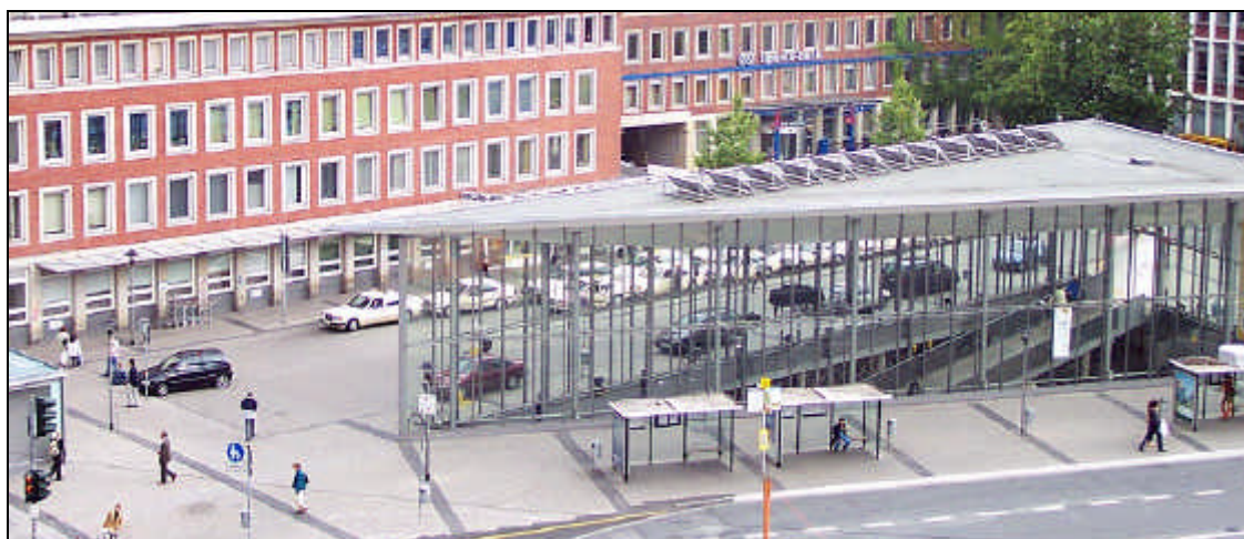
Canopy for underground store immediately outside Münster rail station, Germany. The store extends right under the adjacent 4-lane road.
