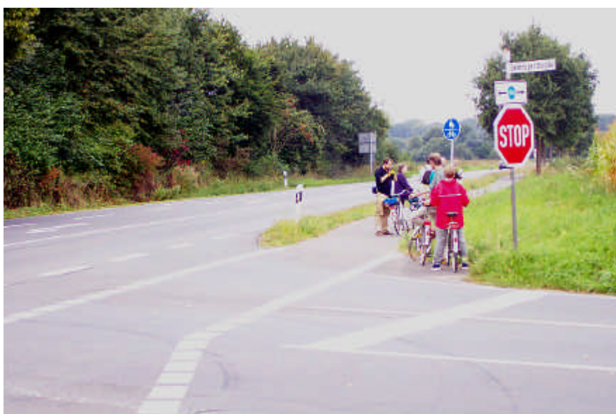
Münster, Germany. (The shared footway descends gradually to road level to cross the side road).
