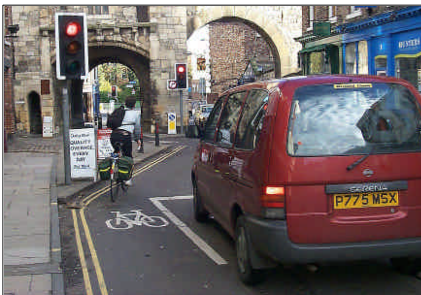
Cyclists are permitted to pass this signal at red simply by virtue of the absence of the stop line. Monk Bar, York.
