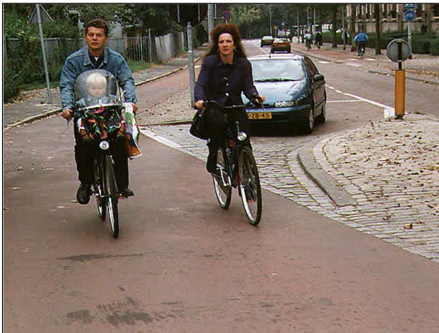
Groningen, Netherlands: vehicles give way to cycles (with appropriately emphatic signing) where the road narrows. The area behind the cyclists is the end of a cycle lane.
